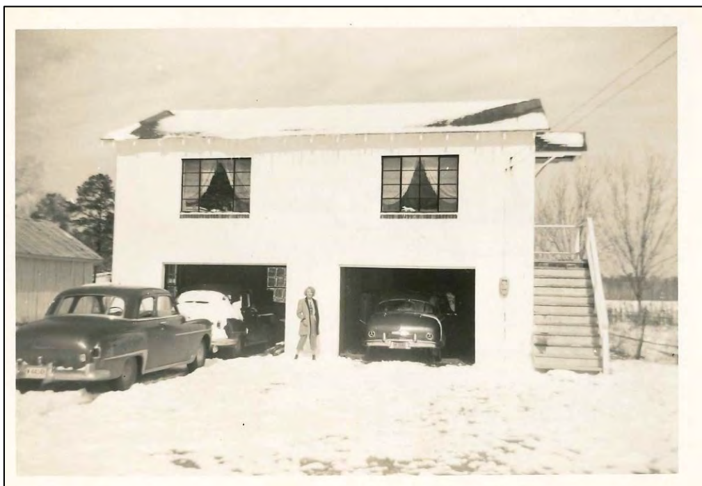
Exhibit 13. Ca. 1950s photograph of the apartment building on the Jesse Trader property, view to the north. The building originally included a two-car garage on the first floor. Note the presence of Outbuilding 3 at frame left. Photo courtesy of Will Lewis.
