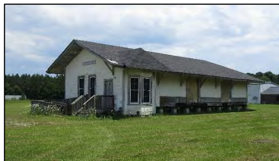
Exhibit 7. Maysville Train Depot, view to the southeast.
