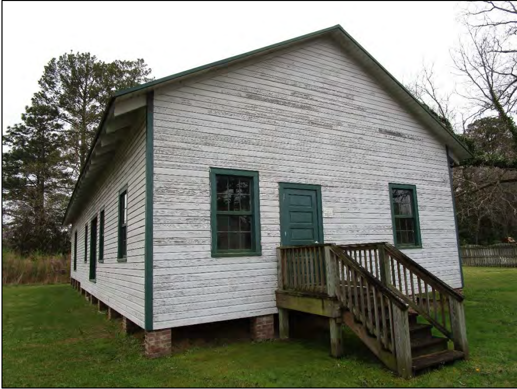
Havelock Station Depot north elevation, view to the southwest.
