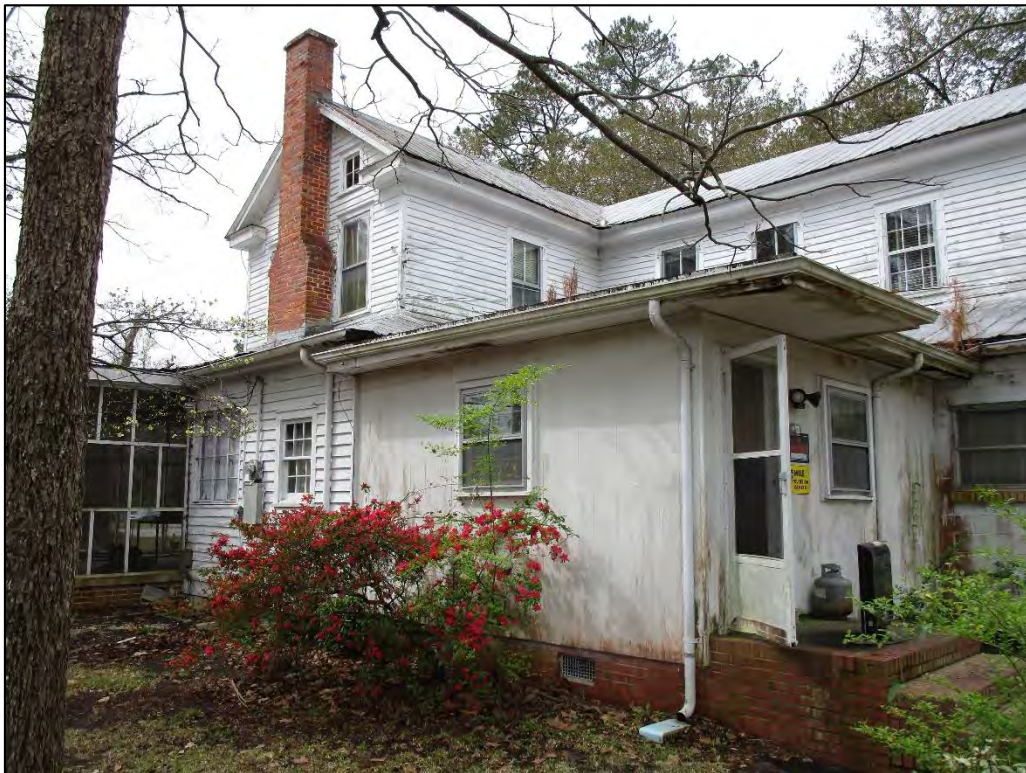
Jesse Trader House oblique view to the southwest; detail of ca. 1980s kitchen addition extending from enclosed wrap-around porch.
