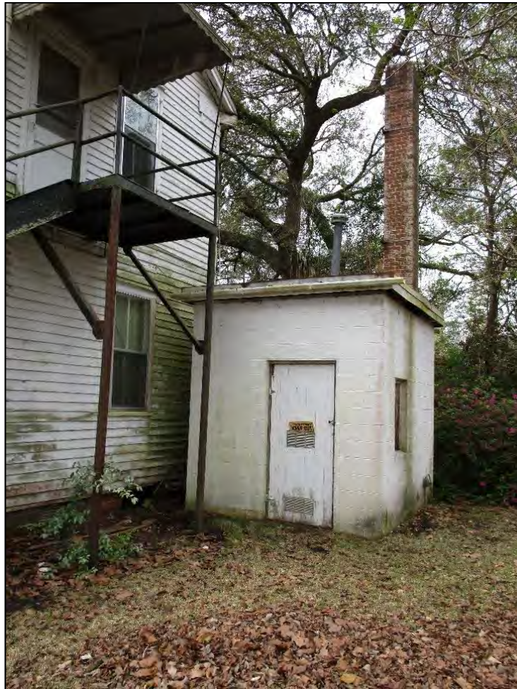
Jesse Trader House, Boiler Room located at the northwest corner of the house; view to the southwest.
