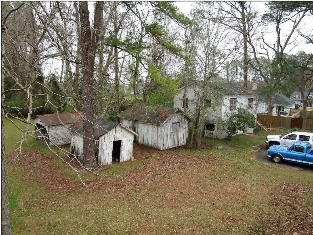
Jesse Trader House, outbuildings and apartment building, elevated view to the northeast.
