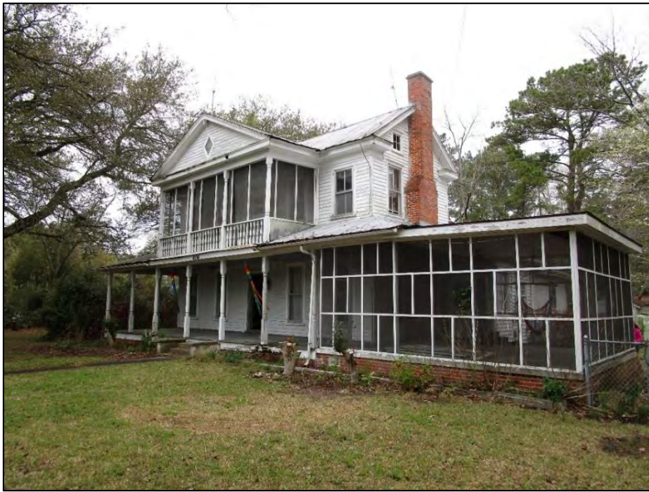
Jesse Trader House façade, view to the northwest
