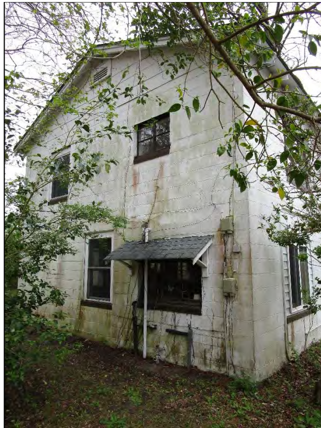
Jesse Trader House, Apartment Building (1950) west elevation, view to the northeast.
