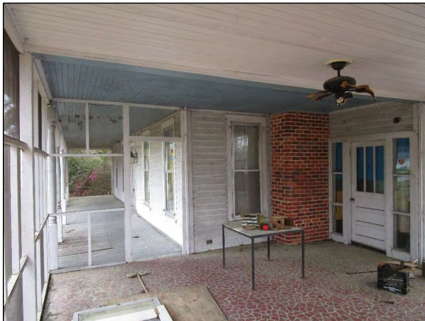
Jesse Trader House; view to the northwest from interior of screened-in porch addition showing the extent of the original wrap-around porch (blue beadboard ceiling), broken tile floor and door addition.
