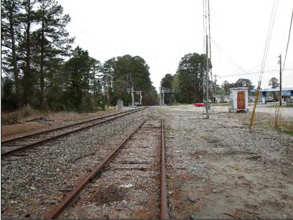
Old Havelock Historic District, view to the northwest from the railroad siding.
