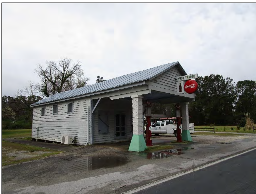
Hugh Trader Store, oblique view of the façade and east elevation, view to the southwest.
