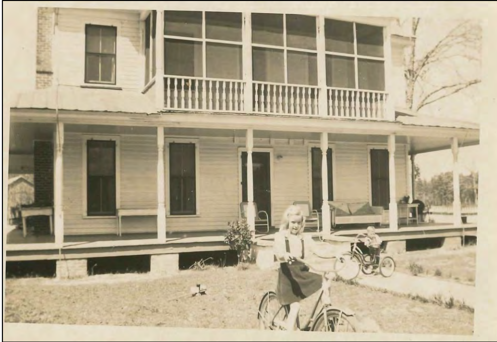
Exhibit 11. Ca. 1930s photograph of the Jesse Trader House, view to the northeast. Note the southeast corner of the wrap around porch remains open, as does the brick pier foundation. A raised-seam metal roof is also in place at this time, and appears to have been installed over cedar shingles, as viewed from attic. Photo courtesy of Will Lewis.
