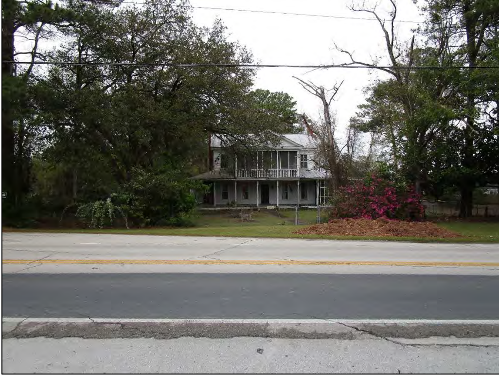
Jesse Trader House façade from the south side of Miller Boulevard, view to the north.
