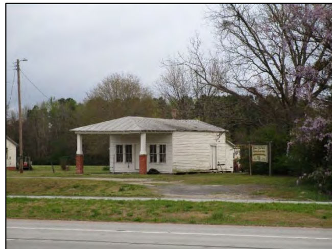
Exhibit 22. The ca. 1920s King Store, contributing structure to the NR-eligible Cobb-King-Humphrey House; view to the northwest.
