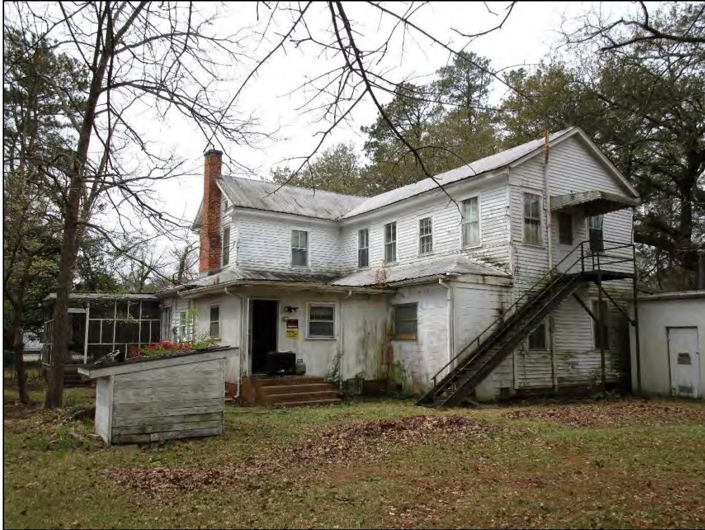
Jesse Trader House oblique view to the southwest of the rear (north) and east elevations.
