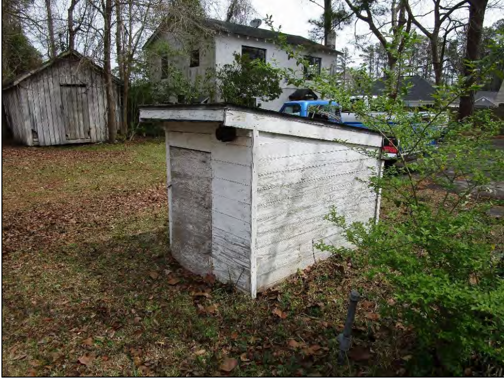
Jesse Trader House Well House, view to the northeast. Outbuilding 3 (left) and apartment building (right) in background.
