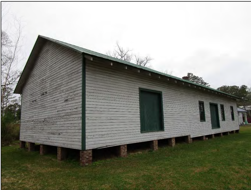
Havelock Station Depot oblique view of the south and east elevations, view to the northwest.
